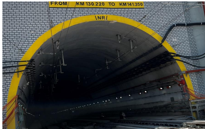
Tunnel T - 41, KRCL
