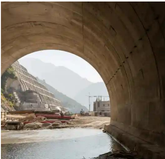
Tunnel T - 5, KRCL
