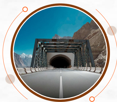
Precast Cut-and-Cover Tunnel, Leh, Ladakh India's Longest Precast Cut-and-Cover Tunnel – Leh, Ladakh
